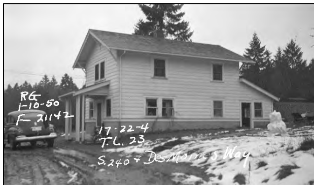
Fig. 16 – These King County tax assessor photos record buildings no longer on the Masonic Home property.
