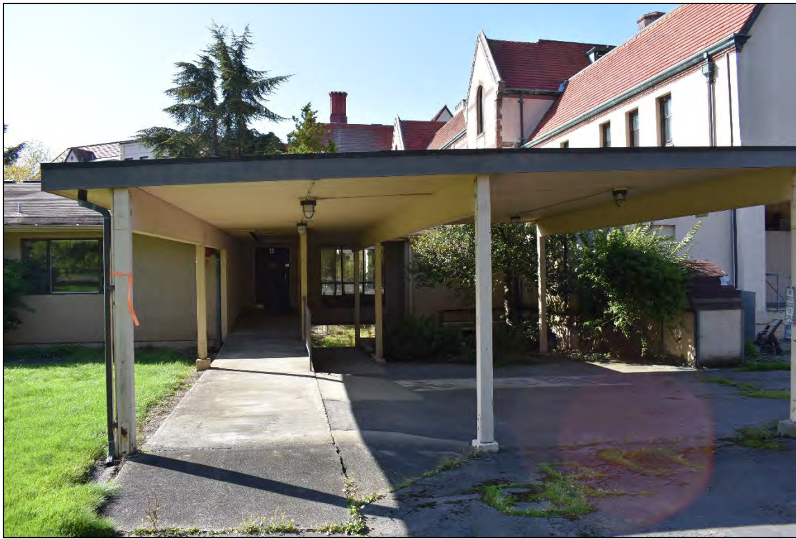
Fig. 26 – Infirmary Wing north arm, east facade, covered entrance. (2019)
