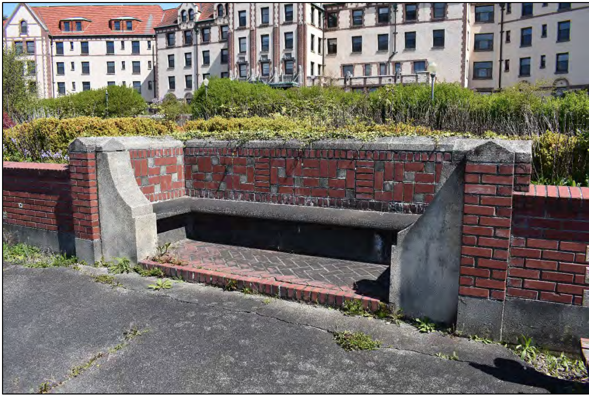
Fig. 101 – Central Oval, brick retaining wall, detail of seating.
