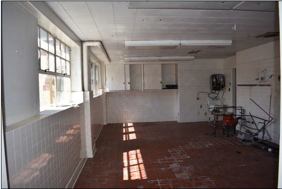
Fig. 52 – Main Building, interior, first floor, kitchen, support space.
