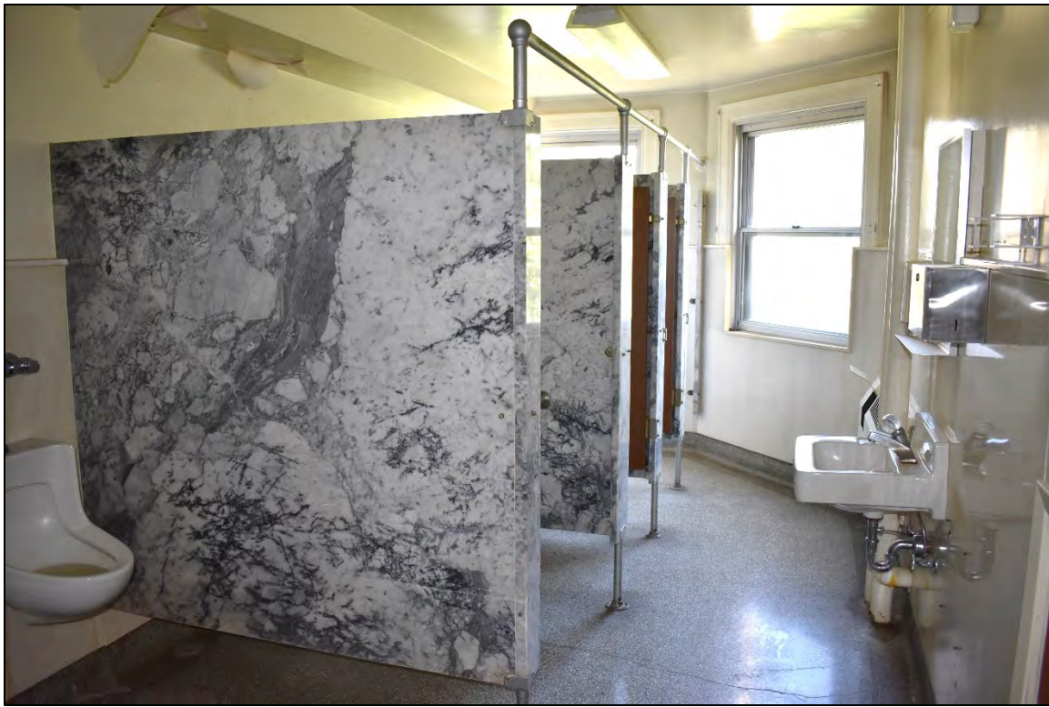
Fig. 75 – Main Building, interior, upper floor, typical shared toilet room.
