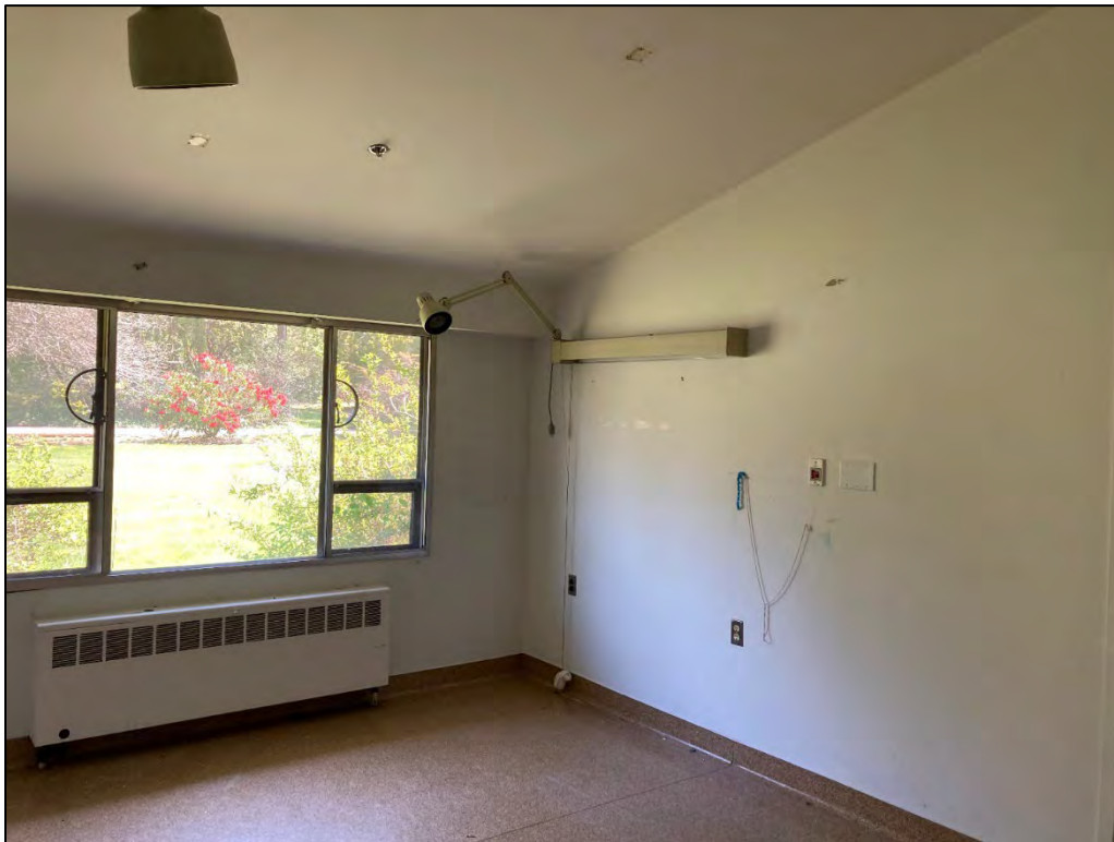
Fig. 92 – Infirmary Wing, interior, first floor, typical ward along corridor (built 1966).
