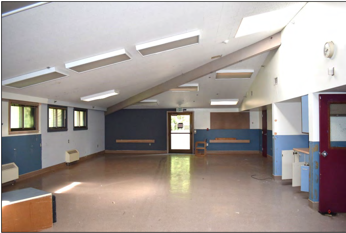
Fig. 95 – Infirmary Wing Addition, interior, first floor, view east. (2019)
