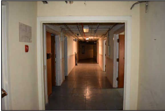
The Basement in 2022
