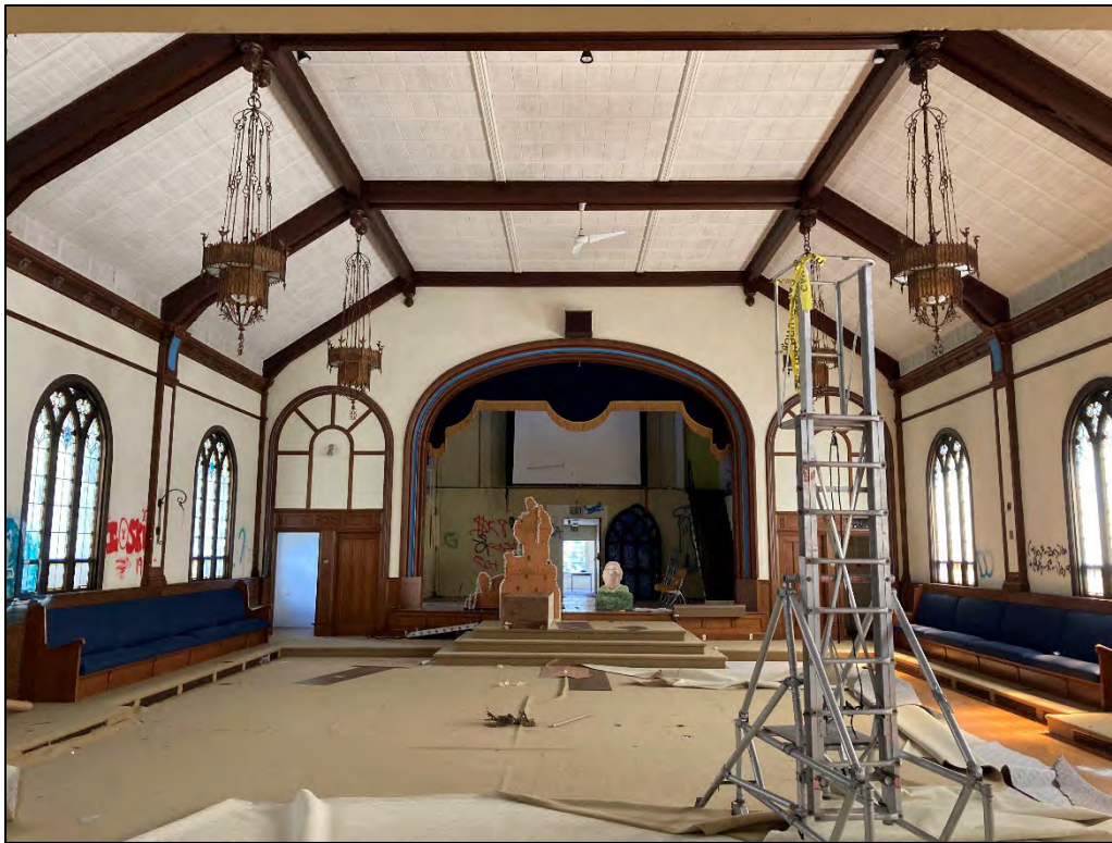
Fig. 57 – Main Building, interior, second floor, chapel/auditorium, view east to front.
