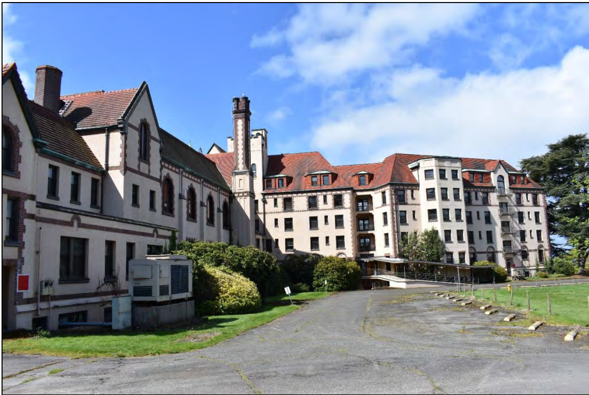
Fig. 12 – Main Building, view west to west facade of north wing (right) and north facade of rear wing (left).
