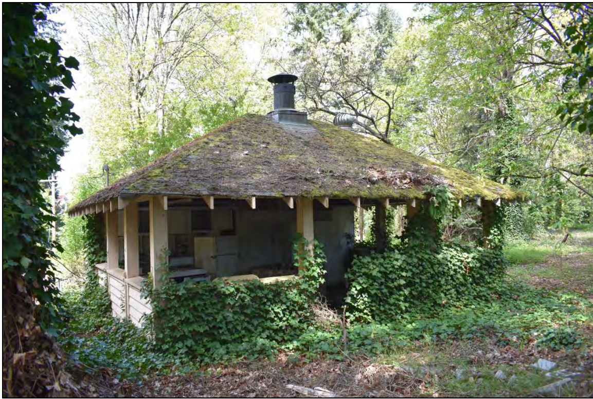
Fig. 115 – Outdoor Kitchen (unknown construction date, mid-20 th century) in woods east of the Main Building.
