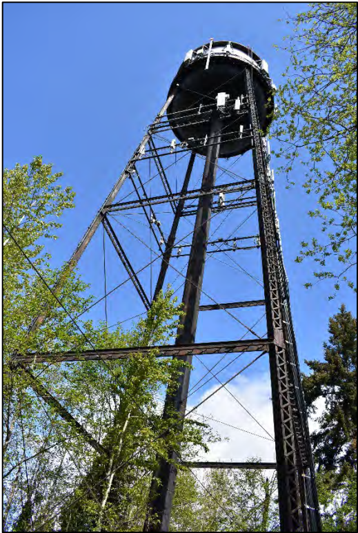
Fig. 112 – Water Tower (built 1926).
