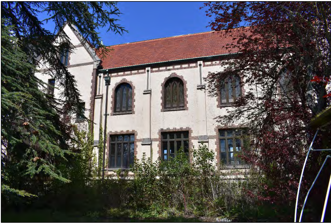
Fig. 20 – Main Building, rear wing, south facade from interior courtyard.
