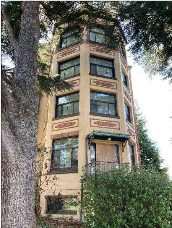
Fig. 11 – Main Building, north wing, north facade (north solarium bay).
