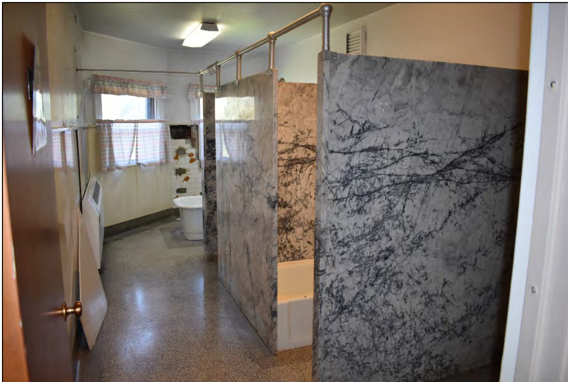
Fig. 74 – Main Building, interior, upper floor, typical shared bathroom. (2019)
