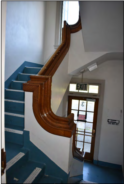
Fig. 56 – Main Building, interior, typical secondary stair. (2019)
