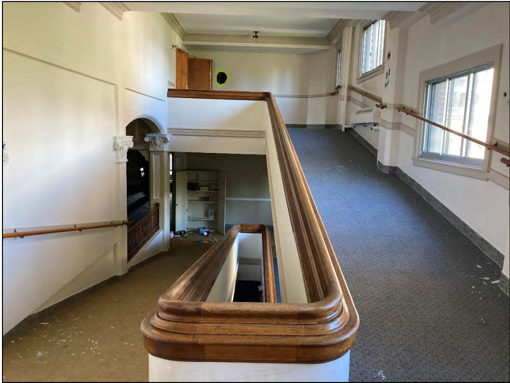
Fig. 54 – Main Building, interior, second floor, main circulation ramps.
