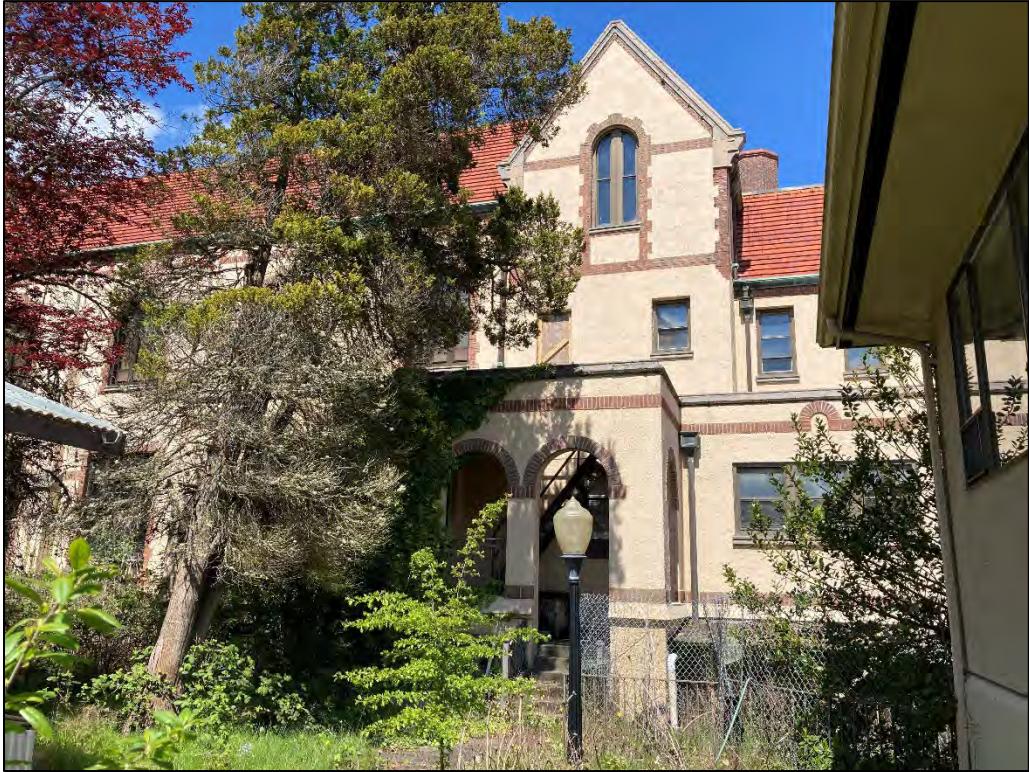
Fig. 19 – Main Building, rear wing, south facade from interior courtyard.
