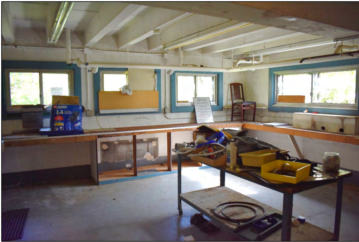
Fig. 79 – Main Building, interior, basement, typical room, showing concrete floor structure overhead. (2019)
