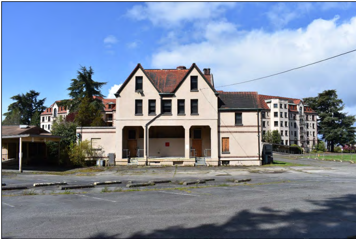
Fig. 16 – Main Building, rear wing, east facade, showing loading dock.
