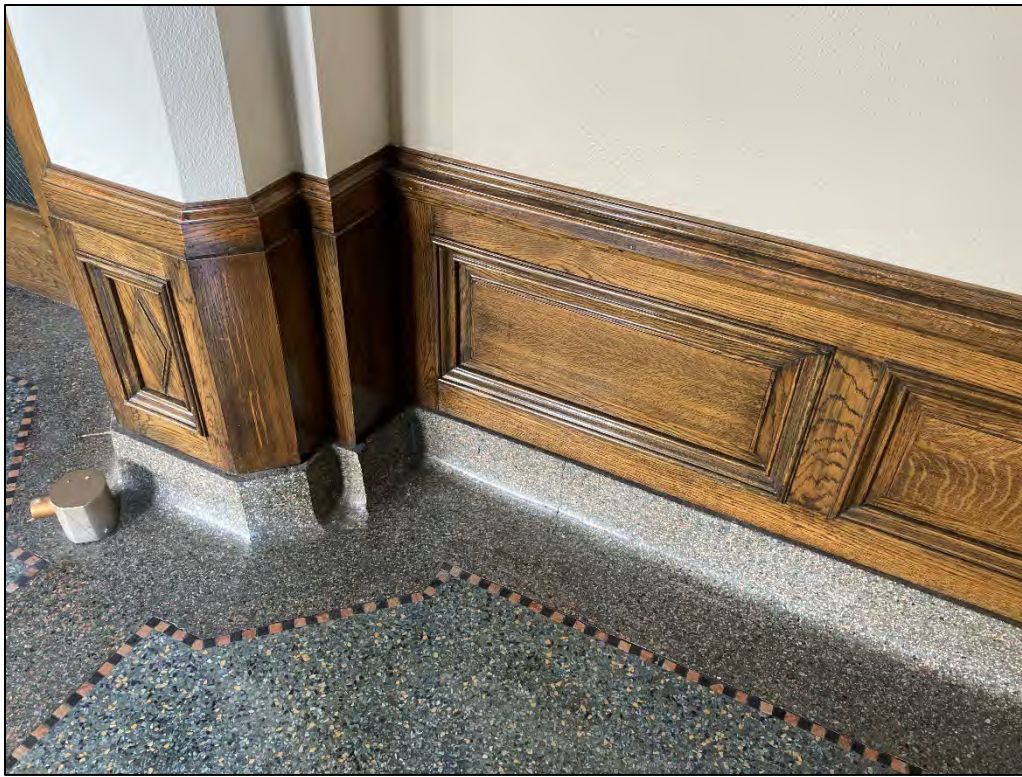
Fig. 41 – Main Building, interior, first floor, main hall, detail of terrazzo floor and wainscoting.
