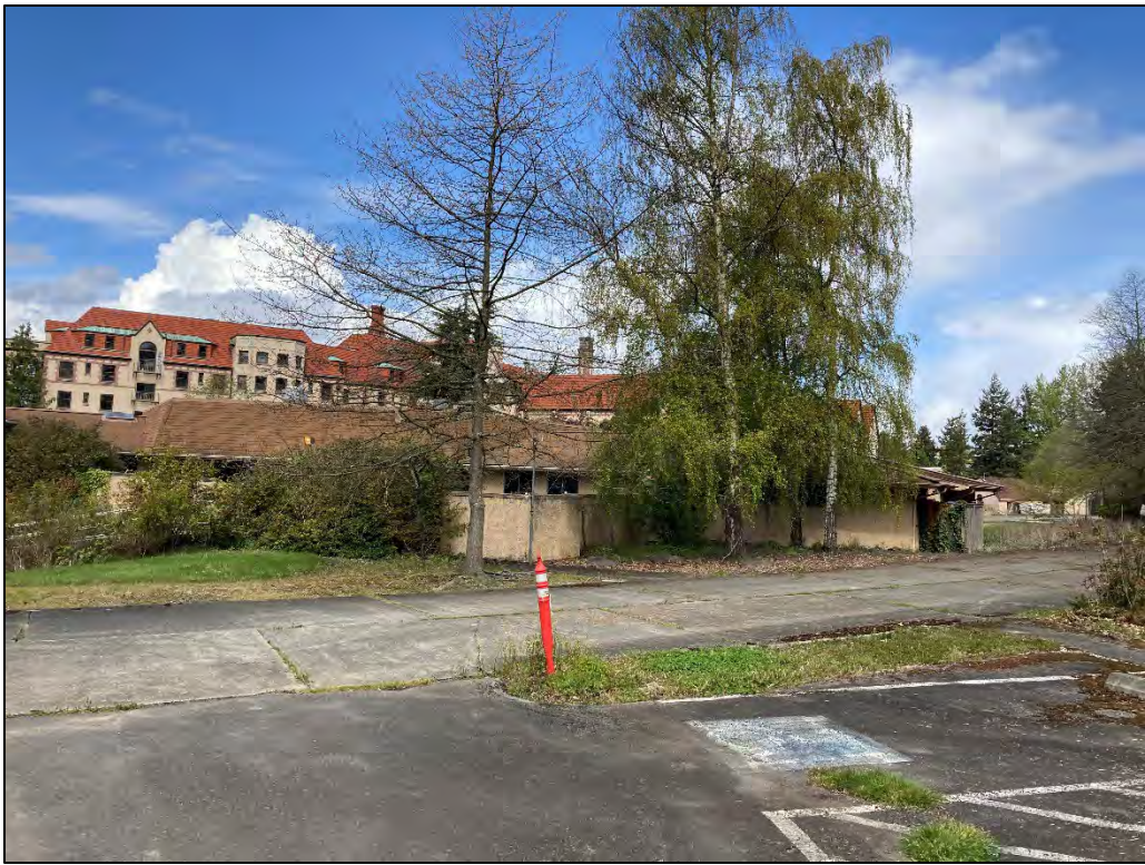
Fig. 28 – Infirmary Wing Addition, east facade.
