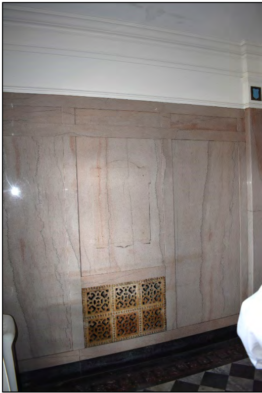
Fig. 39 – Main Building, interior, first floor, entry vestibule. (2019)
