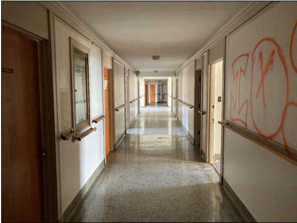
Fig. 66 – Main Building, interior, upper floor, typical residential wing corridor.
