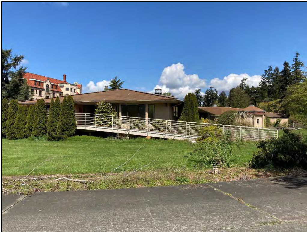
Fig. 33 – Infirmary Wing Addition, southwest facade. Octagonal Pumphouse visible in distance at right.
