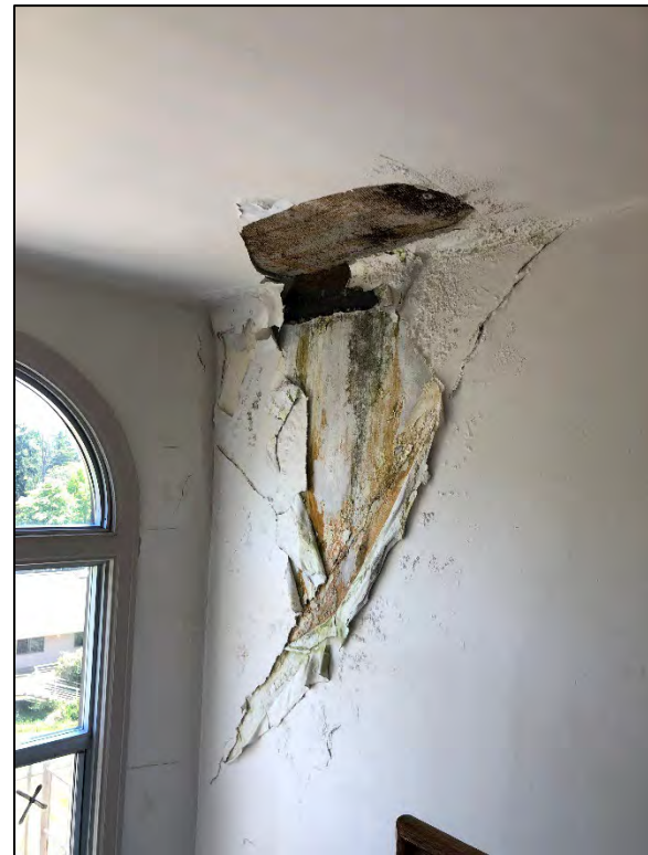
Fig. 90 – Condition: Main Building, interior, fifth floor, water damage at south stair tower
