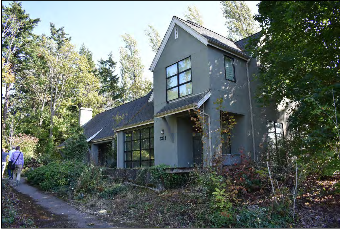
Fig. 122 – House (built 2004 as a model home and sales office) southeast of Infirmary Wing along south property line, view southeast. (2019)
