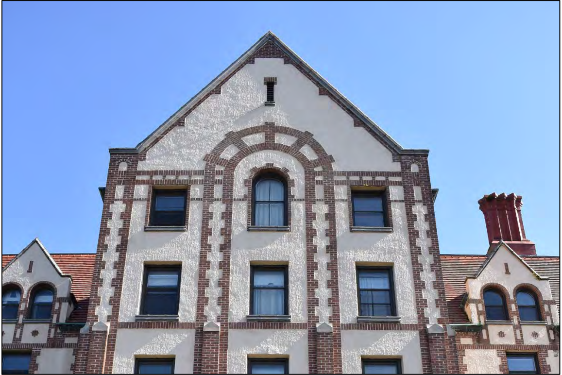
Fig. 5 – Main Building, west facade, detail of central upper gable. (2019)
