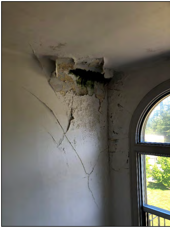
Fig. 89 – Condition: Main Building, interior, fifth floor, water damage at north stair tower
