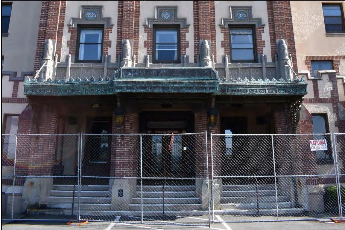
Fig. 37 – Main Building, front entrance. (2019)
