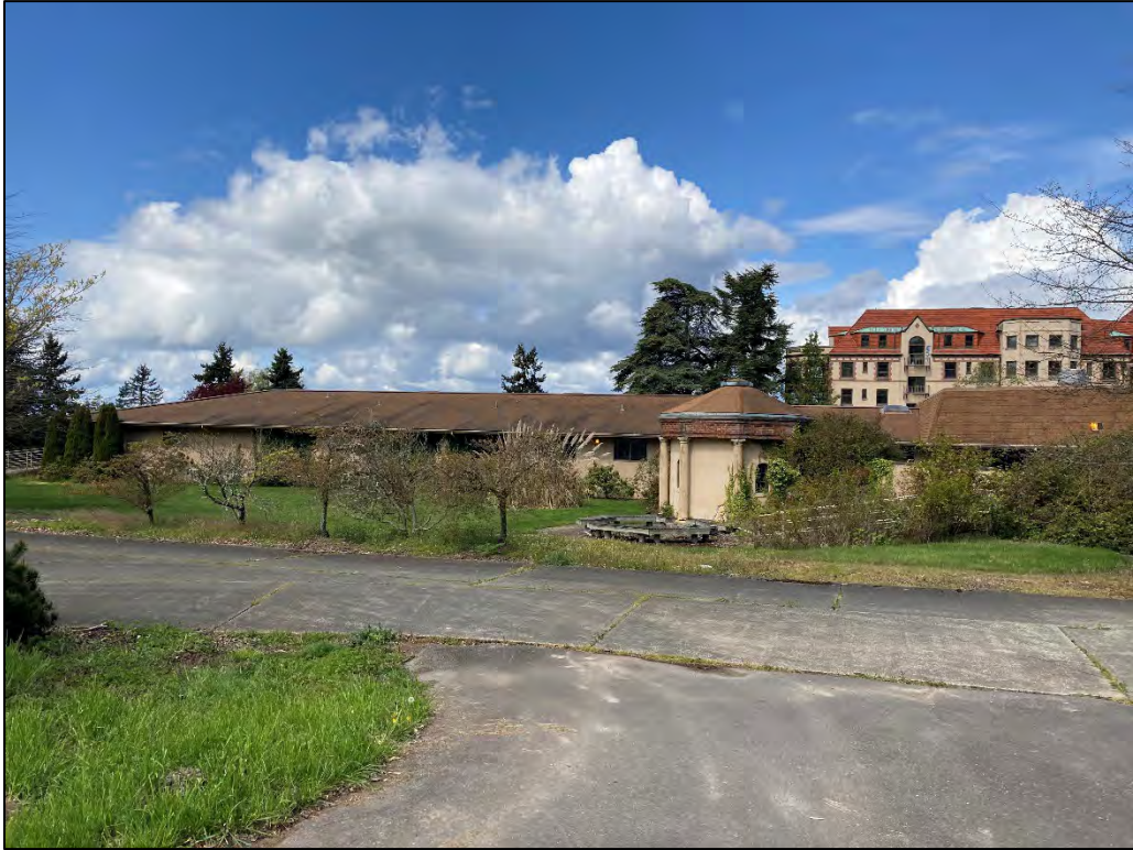
Fig. 29 – Infirmary Wing Addition, east facade. Octagonal Pumphouse visible in foreground.
