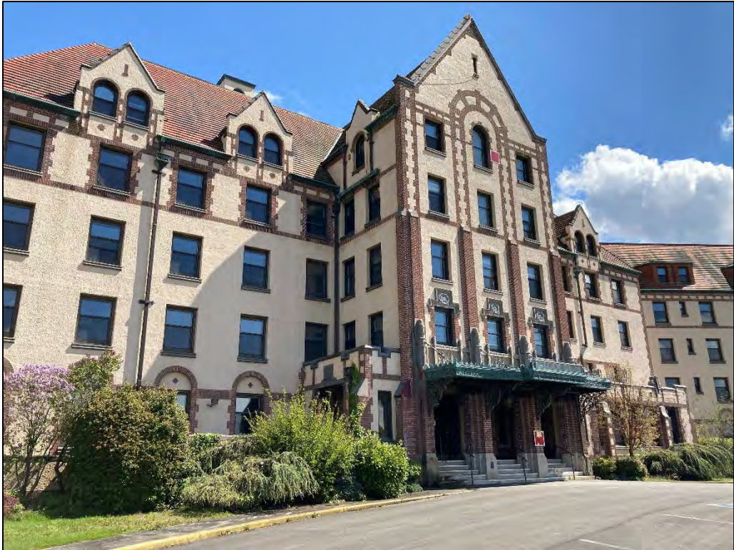
Fig. 3 – Main Building, west facade.
