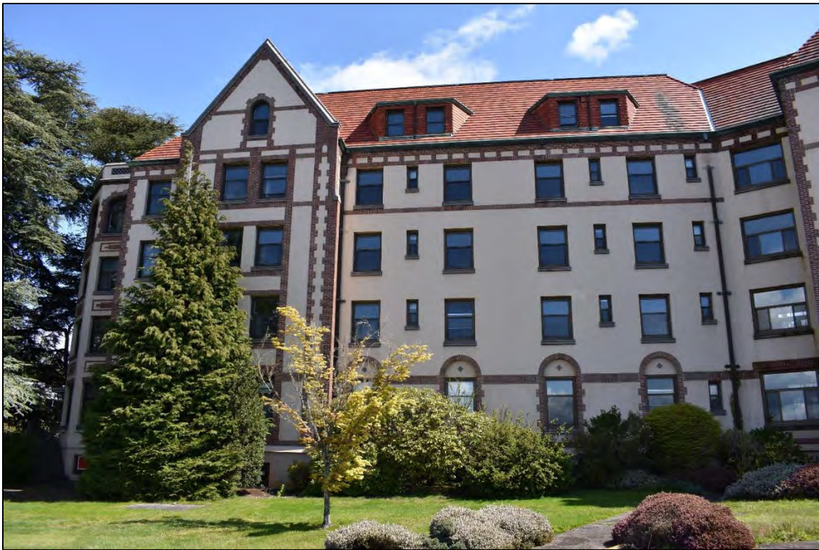
Fig. 10 – Main Building, north wing, west facade.
