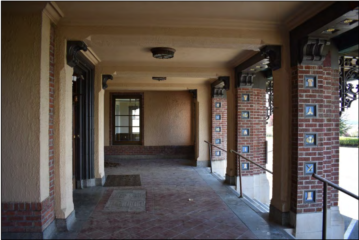
Fig. 7 – Main Building, west facade, main entrance porch.
