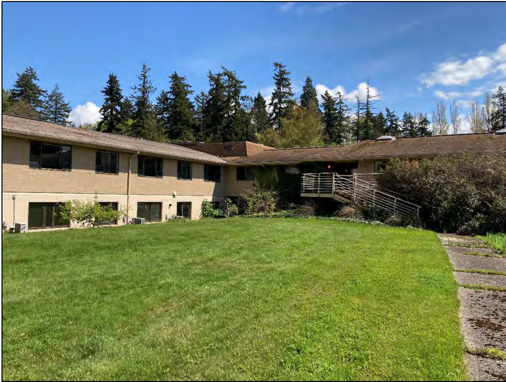
Fig. 35 – Infirmary Wing west arm, southwest facade (left), and Infirmary Wing Addition, northwest facade (right).
