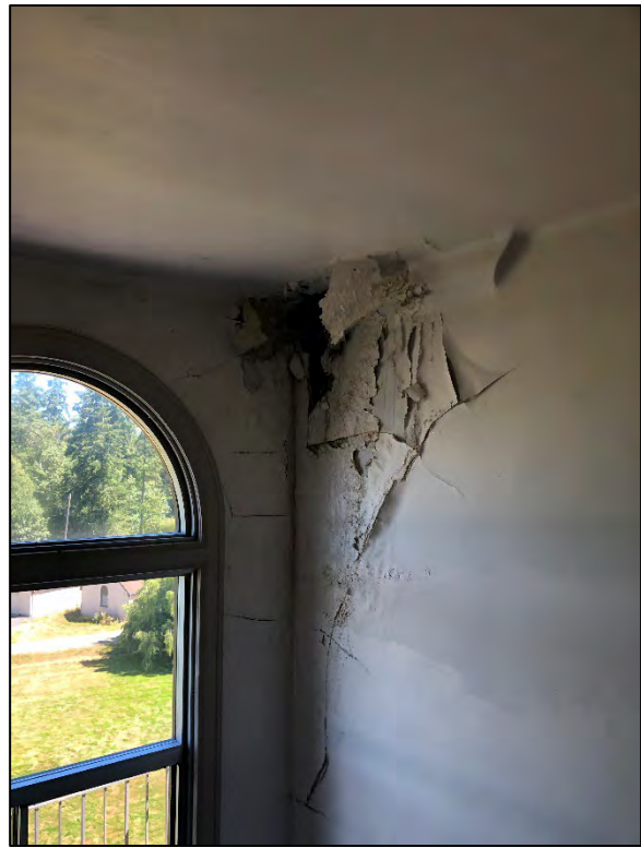
Fig. 89 – Condition: Main Building, interior, fifth floor, water damage at north stair tower
