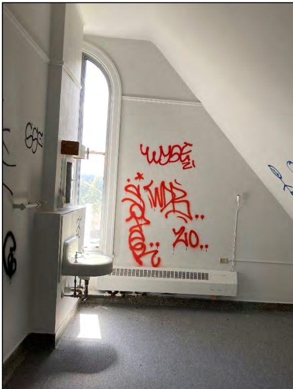
Fig. 70 – Main Building, interior, upper floor, typical residential unit.
