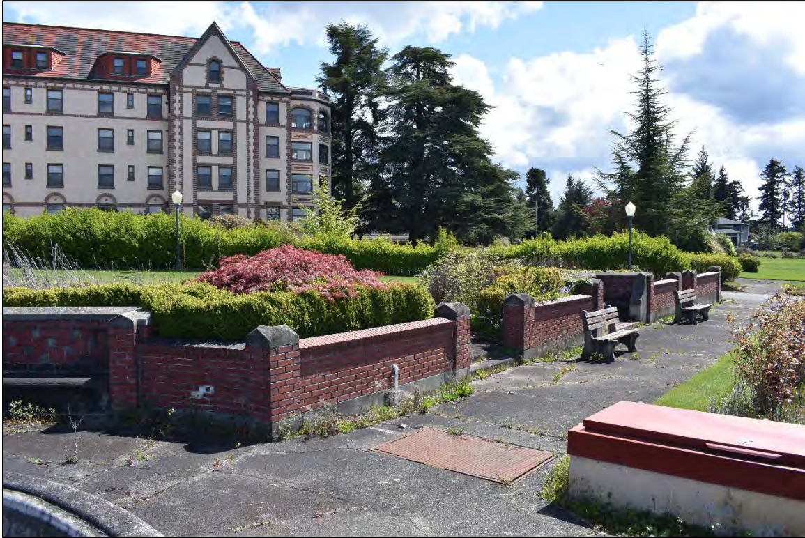
Fig. 100 – Central Oval, brick retaining wall at walk, view south.
