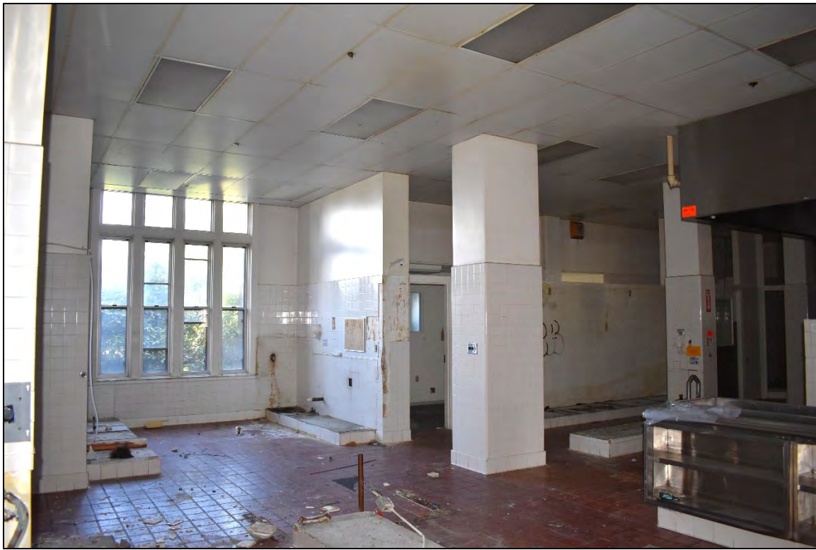
Fig. 51 – Main Building, interior, first floor, kitchen.
