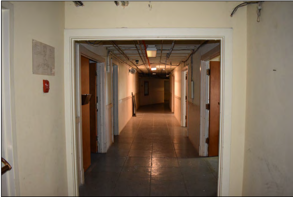
Fig. 76 – Main Building, interior, basement, typical corridor. (2019)
