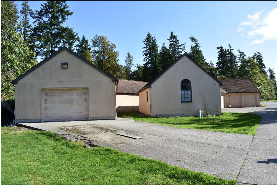
Fig. 114 – Storage Building at left (built 1997); Garage at right (built 1937). (2019)
