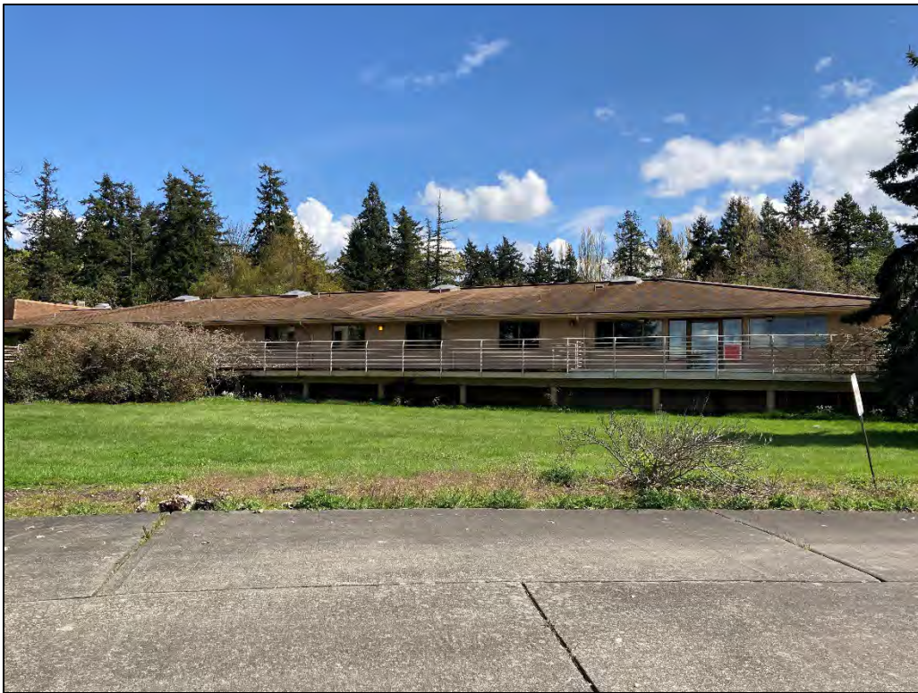
Fig. 34 – Infirmary Wing Addition, northwest facade.
