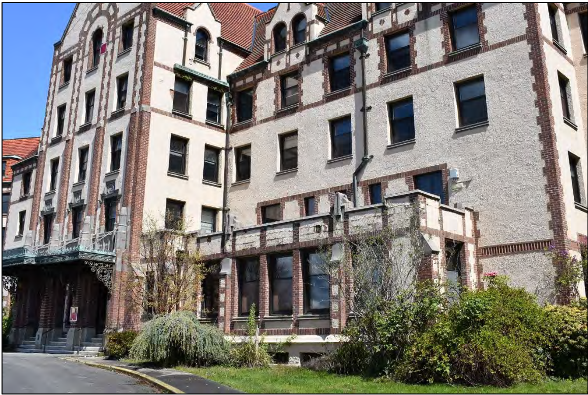
Fig. 4 – Main Building, west facade.
