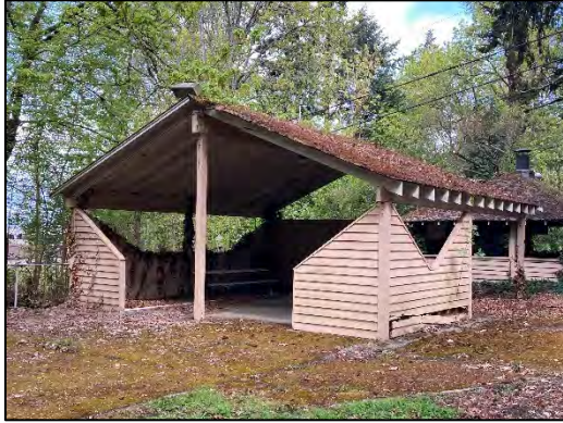
The Covered Patio in 2022
