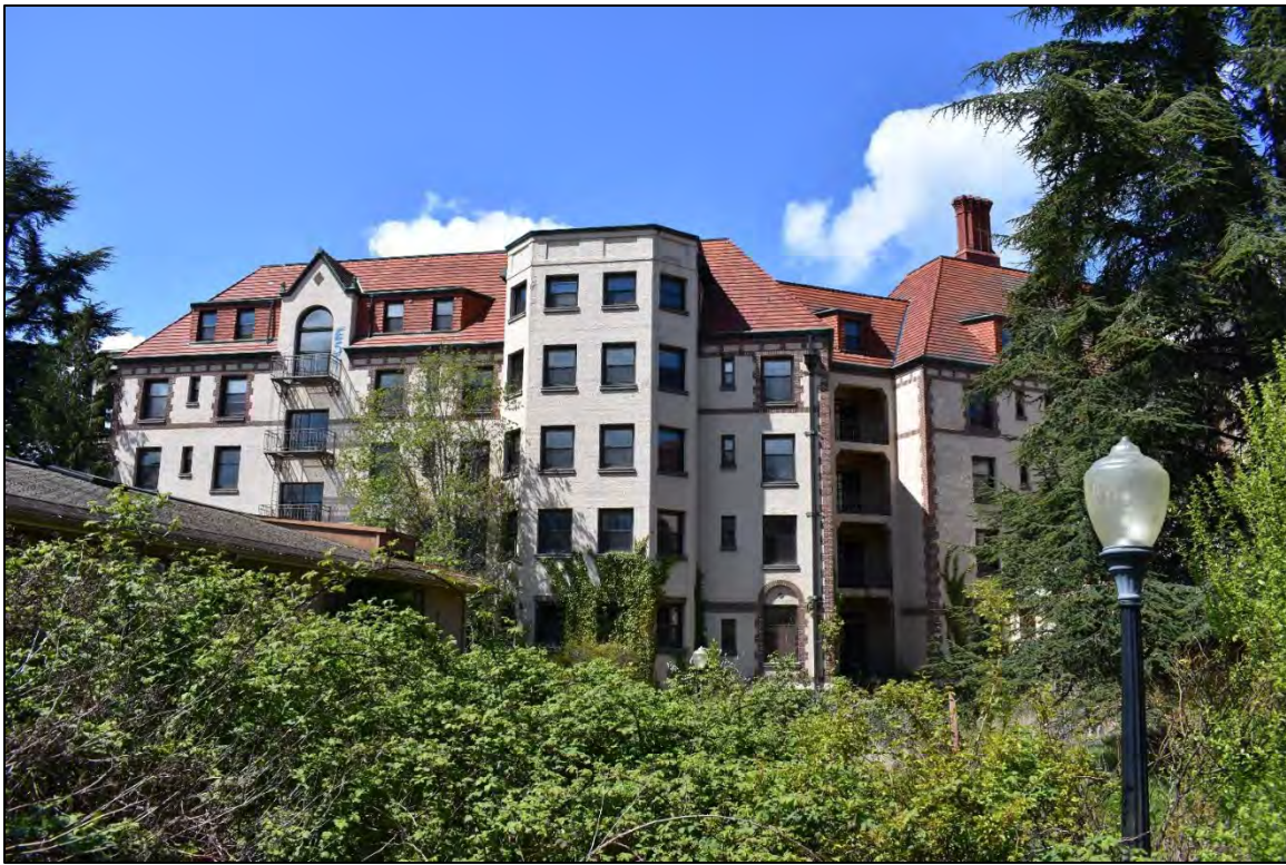
Fig. 22 – Main Building, south wing, east facade, from interior courtyard.
