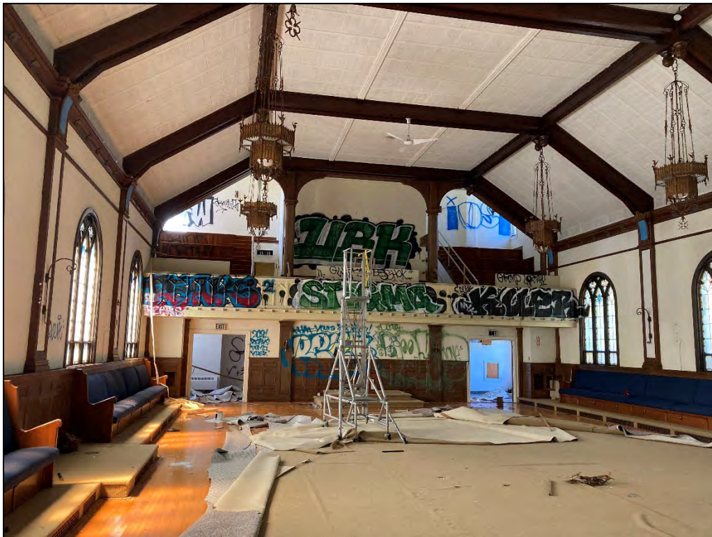
Fig. 58 – Main Building, interior, second floor, chapel/auditorium, view west to rear.
