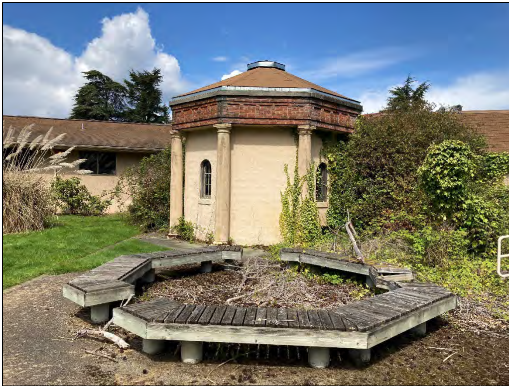
Fig. 32 – Octagonal Pumphouse, east facade.
