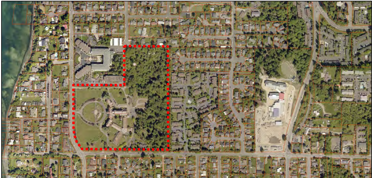
Fig. 7 – Aerial photos of the neighborhood in 1936 and present day.
