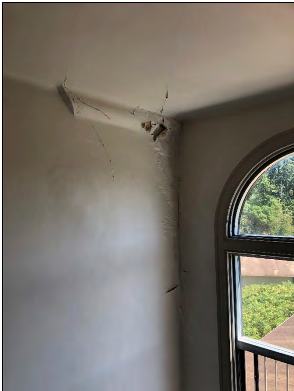
Fig. 90 – Condition: Main Building, interior, fifth floor, water damage at south stair tower
