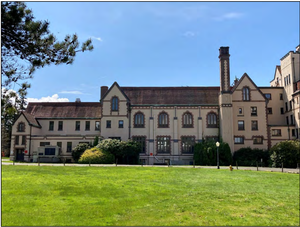
Fig. 14 – Main Building, rear wing, north facade.
