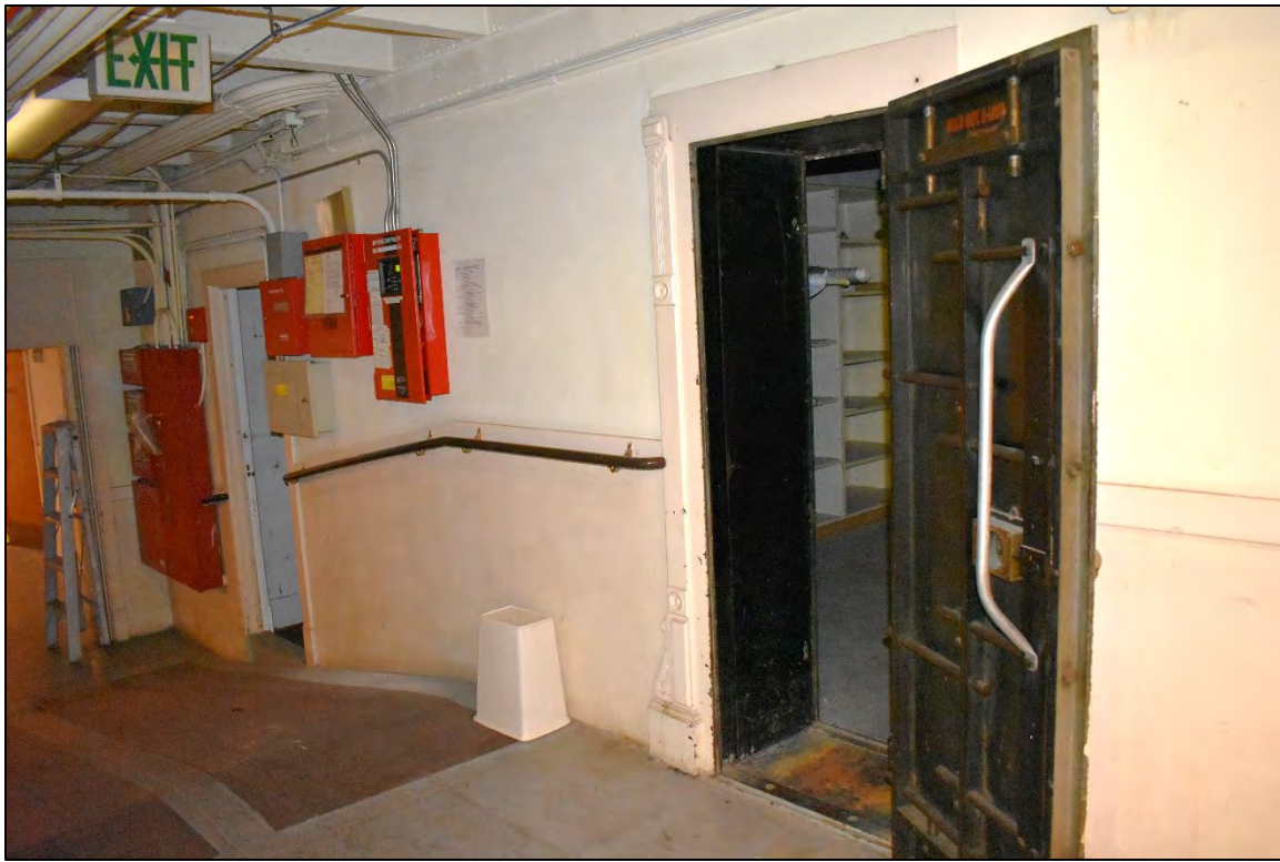
Fig. 77 – Main Building, interior, basement, corridor at vault room. (2019)
