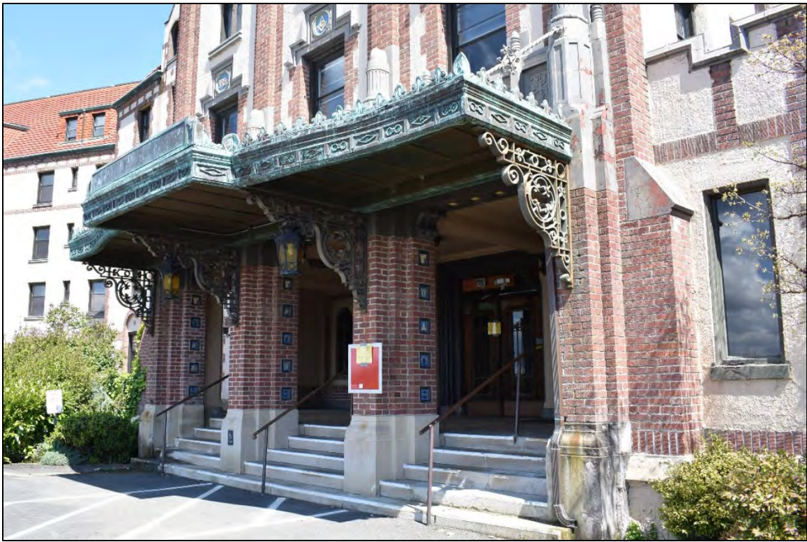
Fig. 6 – Main Building, west facade, main entrance marquee.
