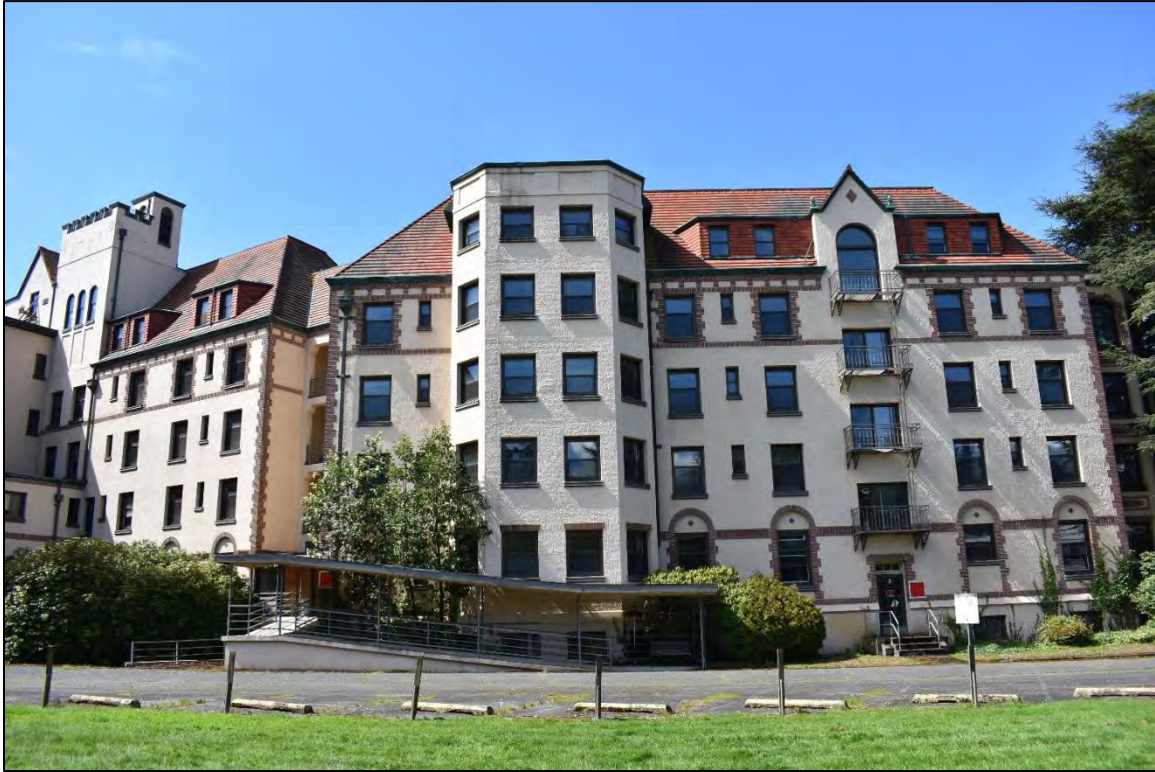
Fig. 13 – Main Building, north wing, west facade.
