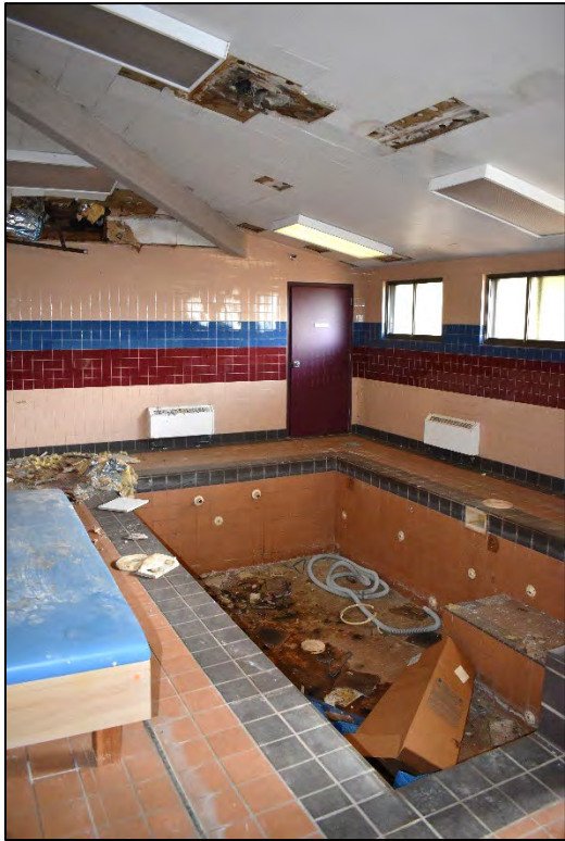
Fig. 96 – Infirmary Wing Addition, interior, first floor, pool therapy room. (2019)
