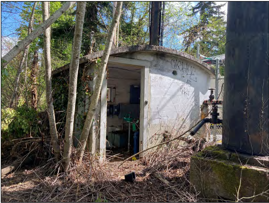
Fig. 113 – Water Tower pump house (built 1926).
