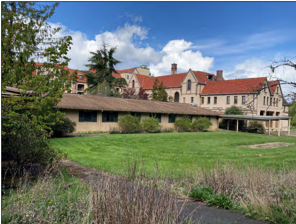
Fig. 17 – Main Building, rear wing (in distance) showing loading dock at right. Infirmary Wing (built 1966) north arm in foreground at left.
