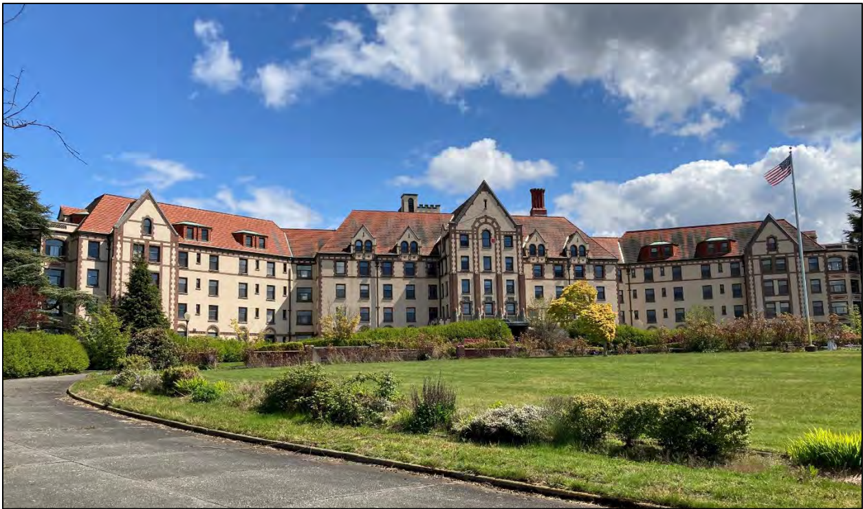
Fig. 2 – Main Building, west facade.
