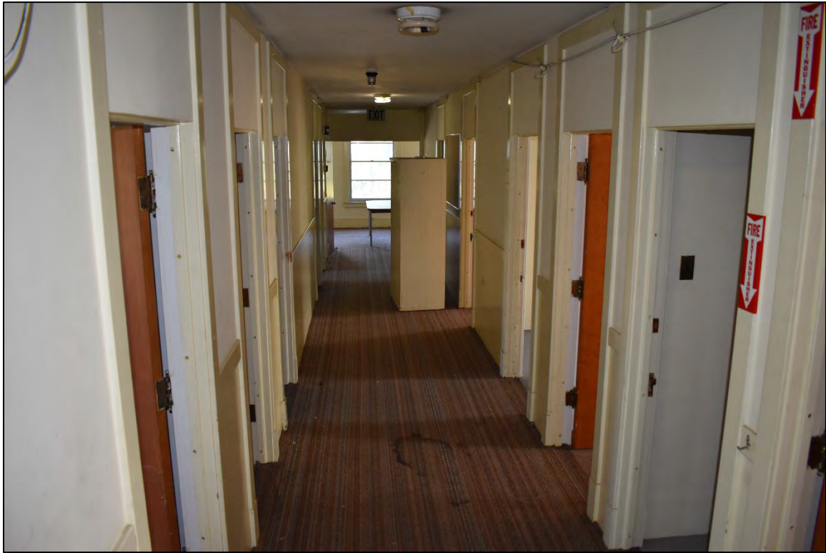
Fig. 62 – Main Building, interior, second floor, dormitory behind chapel/auditorium, view east. (2019)
