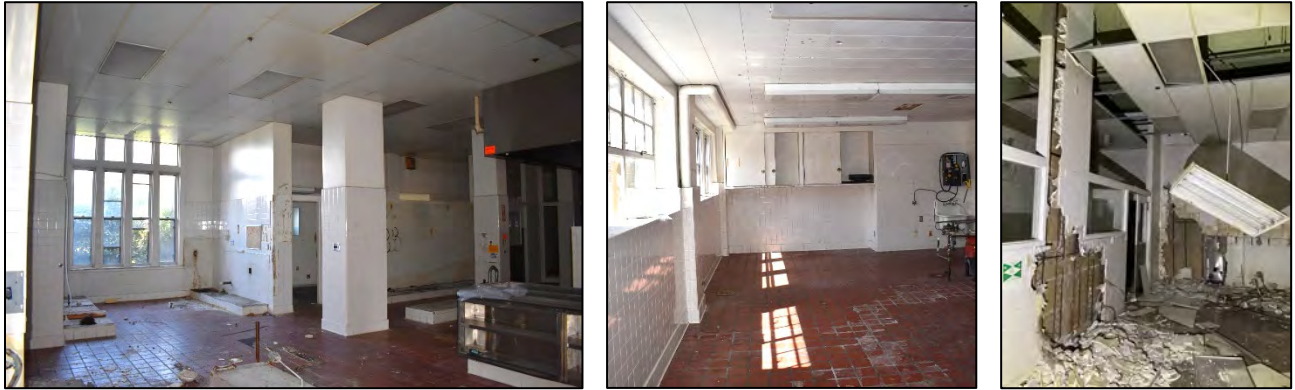
The Kitchen area in 2022 (left and center), and in May 2023 (right)
