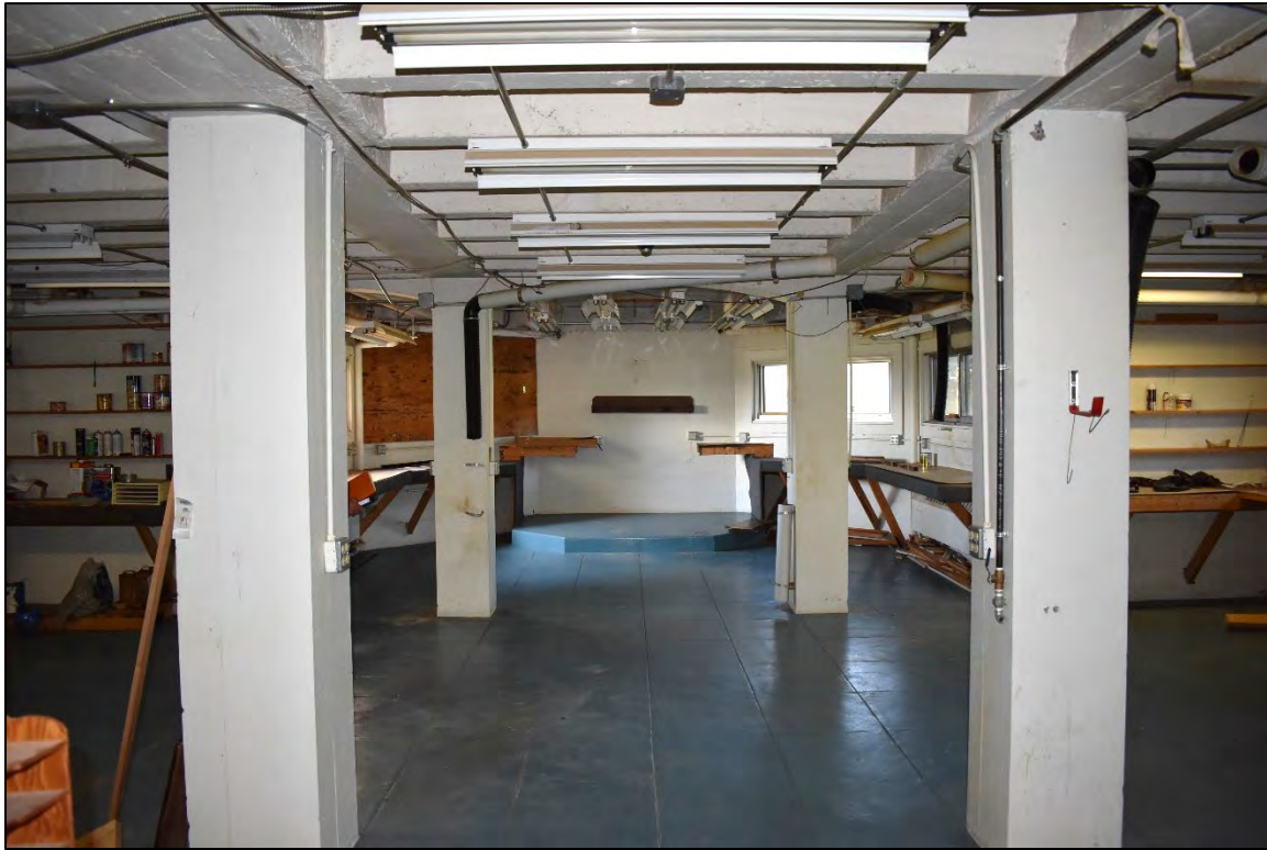
Fig. 78 – Main Building, interior, basement, typical room. (2019)
